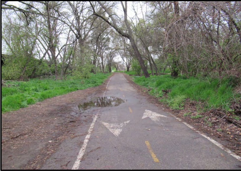
Existing bike path at the east end of the project site, looking northwest; 03/15/21. The proposed bike path will tie into the existing bike path.
